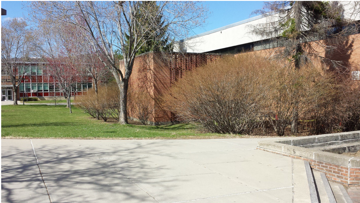
View of mechanical equipment at the Business Building
