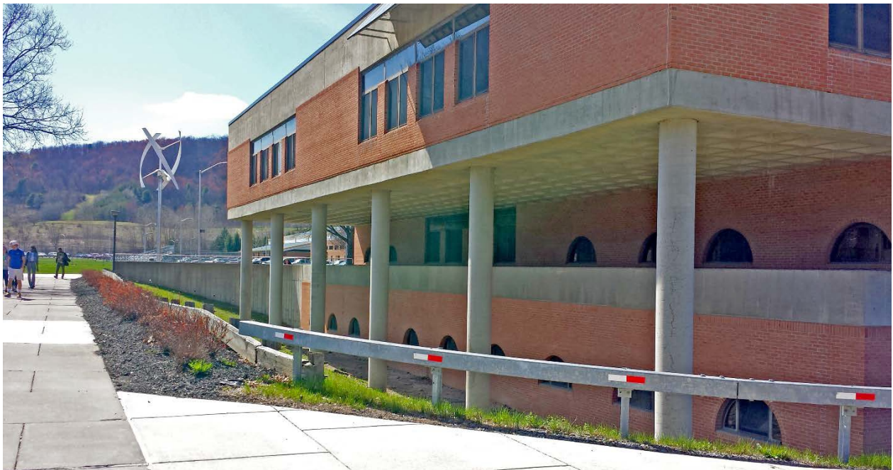
Cantilever over the drainage area, north of the Annex
