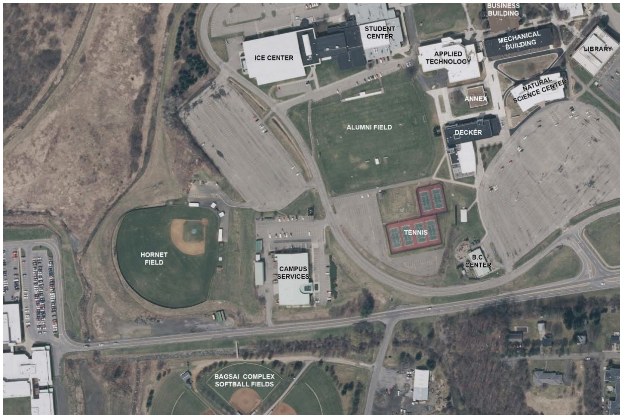
Aerial photo of campus, showing the existing Athletic Facilities
