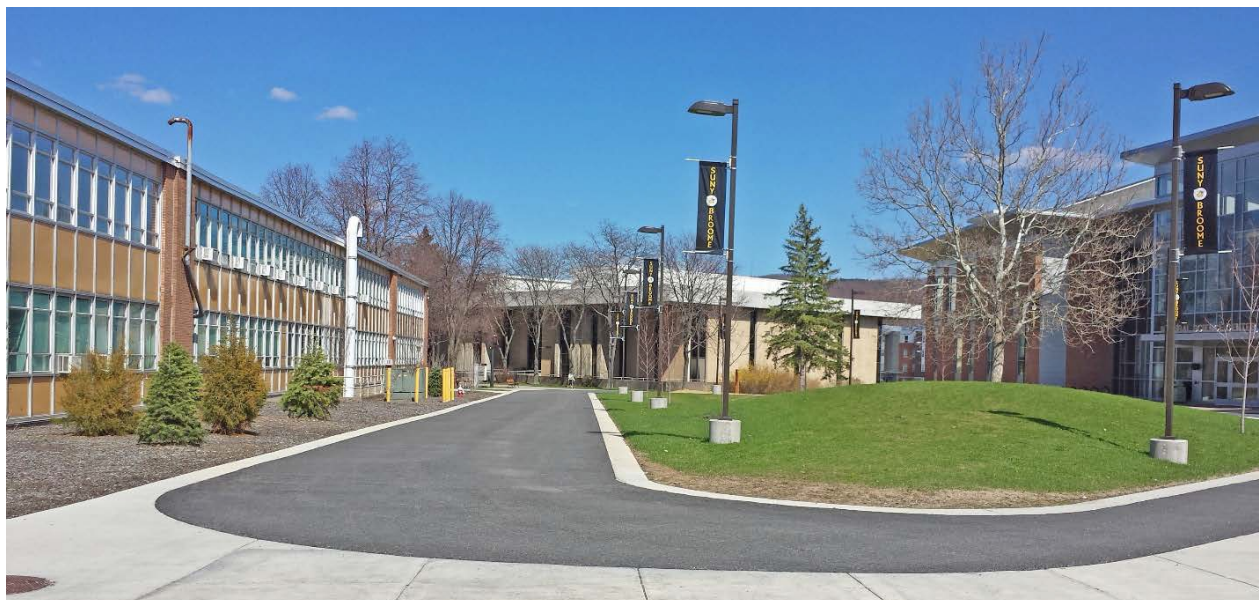
View looking east along the quad toward the Library, showing the lack of entry into the Mechanical Building
